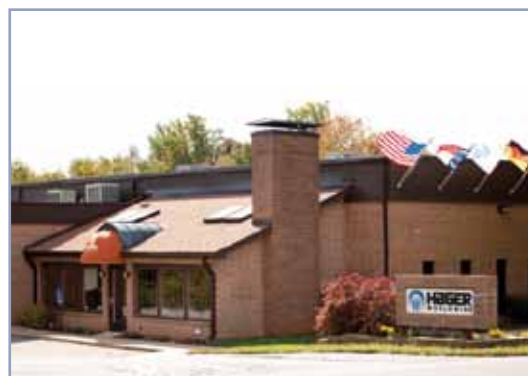
Hager Worldwide Corporate Office Hickory, North Carolina
